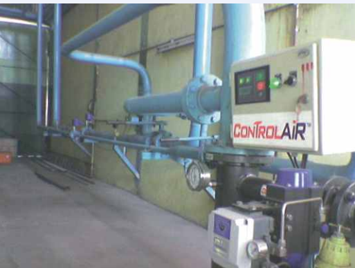
Flow meters for plant air consumption measurement.
