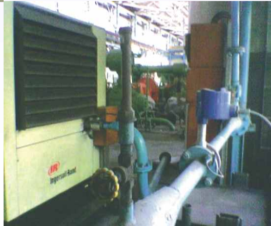
80 mm flow meter for compressor capacity measurement.
