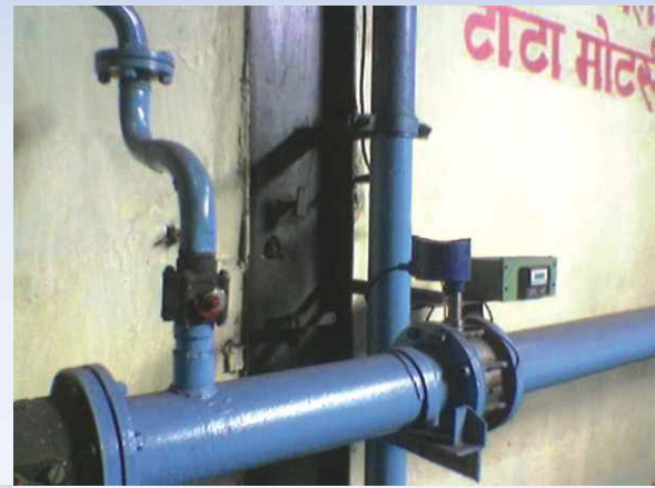
100 mm flow meter in compressed air distribution network.
