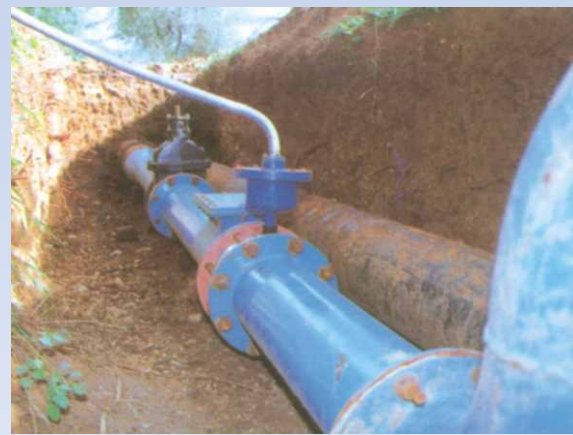
200 mm flow meter for partially flowing gravity pipeline.
