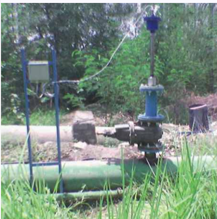
450 mm insertion meter on factory intake water pipeline.
