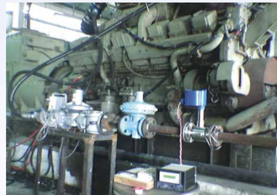
40 mm gas flow meter on engine intake manifold.
