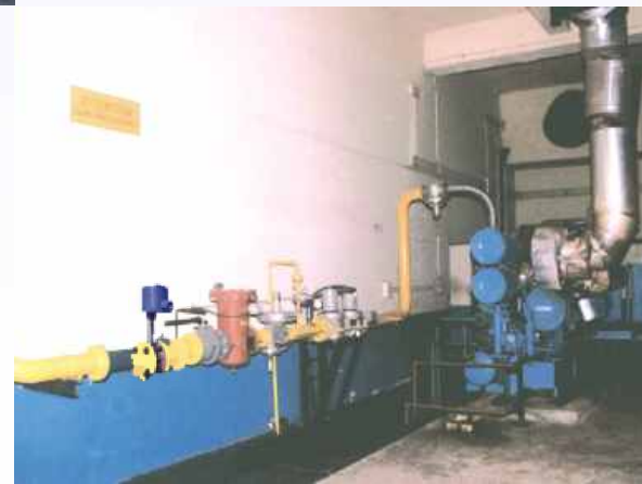
50 mm flow meter on Gas Engine.
